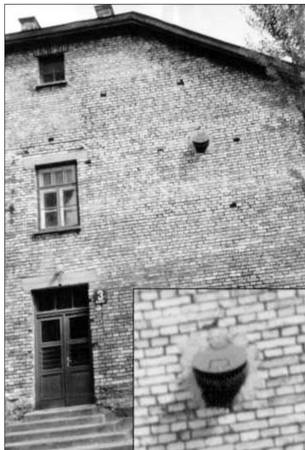
Auschwitz Main Camp, Block 3. Round opening covered by a metal lid, which housed the air-extraction fan for the Zyklon-B fumigation chamber located on the second floor of the building. Enlarged in the inset. (Photo of 1992).
